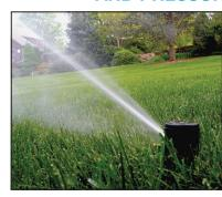
At this point, the system is ready to be tested and adjusted. The water is turned on and piping is tested for leaks. Once we know there are no leaks, the heads are adjusted for proper coverage.
