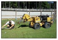
Once your system design is determined we will begin to install the piping. We use a vibratory plow to install the pipe which helps minimize damage to
