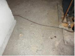
Attention Recommended - The fuel line runs across a pathway in the basement. Damage can occur to the line. Protection or redirecting the fuel line is recommended.
