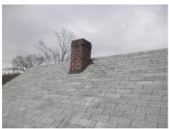
**Action Recommended** - The chimney does not meet the required height. The chimney should extend 3 feet above the roof through which it protrudes or be 2 feet above any surface within 10 feet horizontally, whichever is higher.
