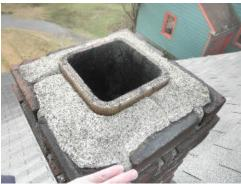
Attention Recommended - The chimney drip cap is made of mortar. Its function is to keep water from entering between the masonry stack and brick, causing deterioration. This cap needs some repair so that it can function as intended.
