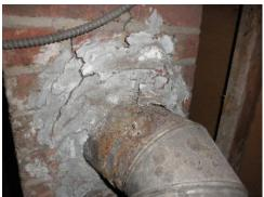
The flue pipe is metal **Attention Recommended**-The furnace/boiler flue as installed appears to need some attention. The boiler stack should be properly sealed to the chimney.
