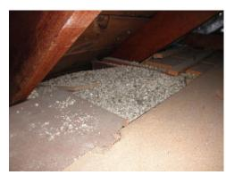
Action Recommended - The some of the insulation in the attic contains vermiculite. Certain brands of vermiculite, manufactured prior to 1990, <a href="mailto:may">may</a> contain asbestos fibers. The date the vermiculite was installed is unknown. Advantage Home Inspections does not perform tests for asbestos.
