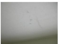
Attention Recommended - There is a condition in the ceiling of the noted room that needs to have attention. There is evidence of an unrepaired stain on the wall caused by a prior moisture leak. Front left bedroom.
