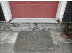
The noted door(s) is located Front, The exterior door in the noted location(s) is: Steel, **Attention Recommended** - The wood frame around the exterior door has water damage at the bottom.
