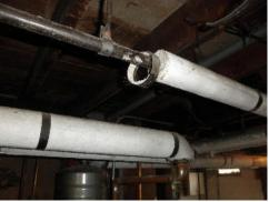
The heat pipes are covered with an insulation which may contain asbestos. Asbestos can only be confirmed by a qualified lab. Advantage Home Inspections does not perform tests for asbestos. **Attention Recommended** - The copper pipes as it connects to the cast iron pipe has signs of deterioration.
