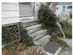
**Action Recommended** - The steps need some repair or replacement. **Action Recommended** - One or both of the hand rails are damaged. Repair is recommended.
