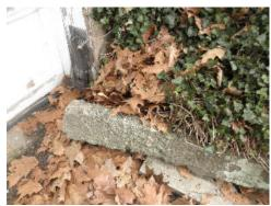
The retaining wall is made of concrete. Partially collapsed.
