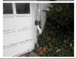
**Attention Recommended** - The gutter system on the roof edge appears to be inadequately sloped to carry the water to the downspouts. Porch gutter Run-off water needs to flow away from the side of the house at least 6 feet. This will allow the run-off to get far enough away to not interfere with the foundation.
