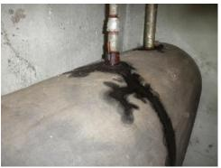
The diameter of the vent pipe is smaller than the fill pipe. This can cause blow back through the tank joints. Replacement is recommended.
