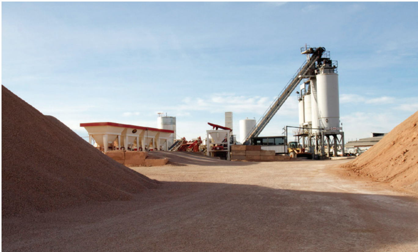
The RAP trend was the biggest reason J & J Asphalt decided to upgrade its 80-tph plant to a RoadBuilder Series, with capacities ranging from 110 to 350 tph.
