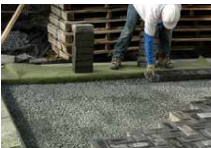
10. Placing the AquaPave® pavers.
