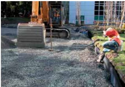
4. Placing and spreading of the clear crushed open-graded upper Sub-base.
