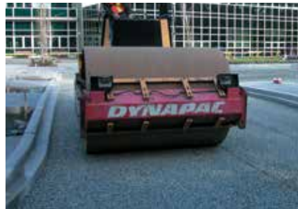
5. Compaction of the clear crushed open-graded upper Sub-base.
