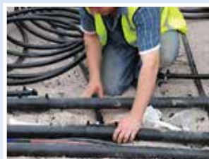
3. Install the geothermal horizontal collector pipes
