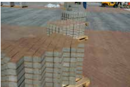
8. AquaPave® pavers are delivered to site, prearranged on pallets .
