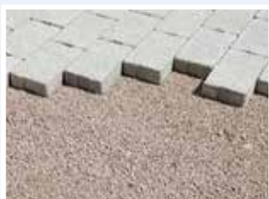
7. Install the AquaPave® pavers
