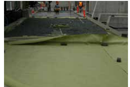
6. Placing the Inbitex® geotextile.
