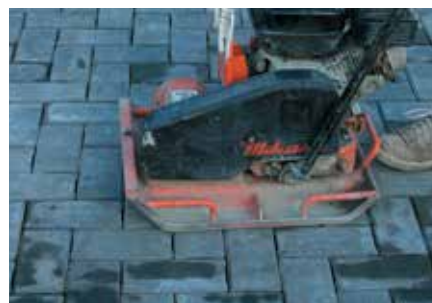
11. Initial compaction of the AquaPave® pavers.
