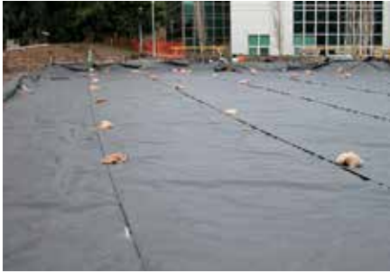
1. Placing the AP SC1000 woven geotextile with the specified overlap.
