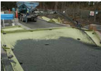
7. Placing and spreading of the 5mm clear crush bedding material.
