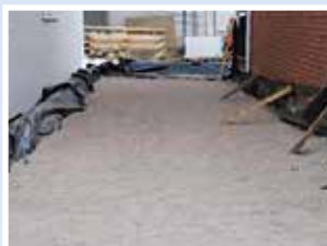
2. Lay and compact 2-6 mm clean bedding stone
