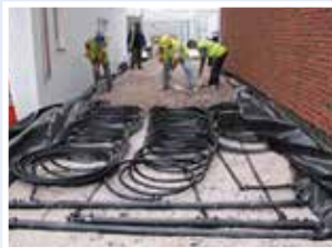
5. Install and compact the graded sub-base stone
