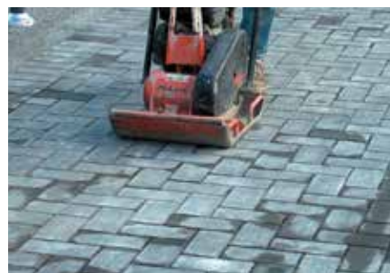
14. Final compaction of the AquaPave® pavers.
