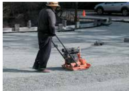
8. Compaction of the 5mm clear crushed open-graded bedding material.
