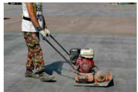
12. After final compaction the paved area is available for immediate use.
