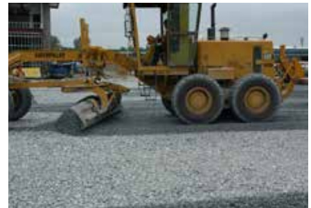
6. Upper Sub-base is then graded to elevation and compacted.
