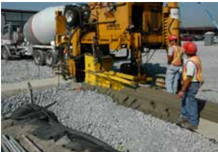
4. Paver restraints are placed.
