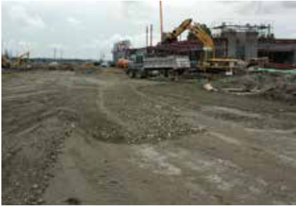
1. Excavation of sub-grade, removing any organic material.
