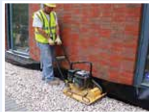
6. Compact for laying course
