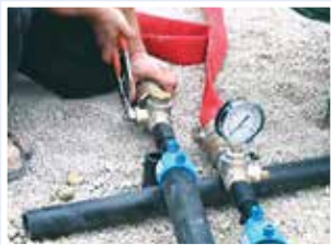
4. Pressurize and system check
