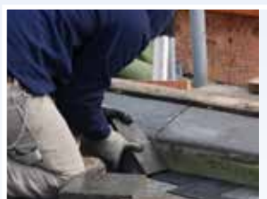
8. Trim Inbitex®, AP SC1000 and SC Membrane® at finished grade
