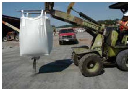
11. AP Engineered Joint Stabilizer is applied and swept into place.
