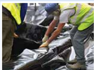
1. Install welded membrane
