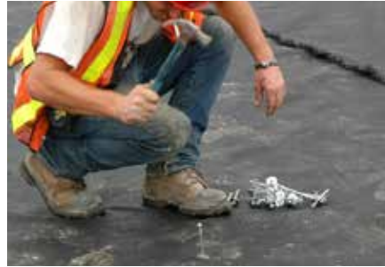
2. AP SC1000 geotextile is rolled out and fastened to sub-grade .
