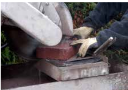
10. All cuts must be made with a masonry saw.
