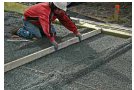
9. Loose screeding of the 5mm clear crush open-graded Bedding Course.
