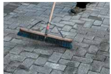
12. Spreading and sweeping in of the AP Engineered Joint Stabilizer.
