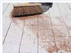
9. Final compaction and sweep in the AP Engineered Joint Stabilizer
