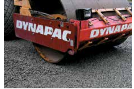
3. Compaction of the lower Sub-base.
